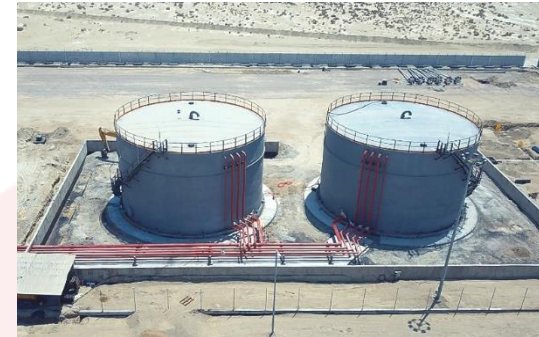
Cooperation in the production and localization of (A516Gr.70 Nace, A283Gr.C Nace sour service) sheets and 6,000 MT of sheets API 5L X60 Nace, API Gr.B Nace of storage tanks of Goreh-Jask .
